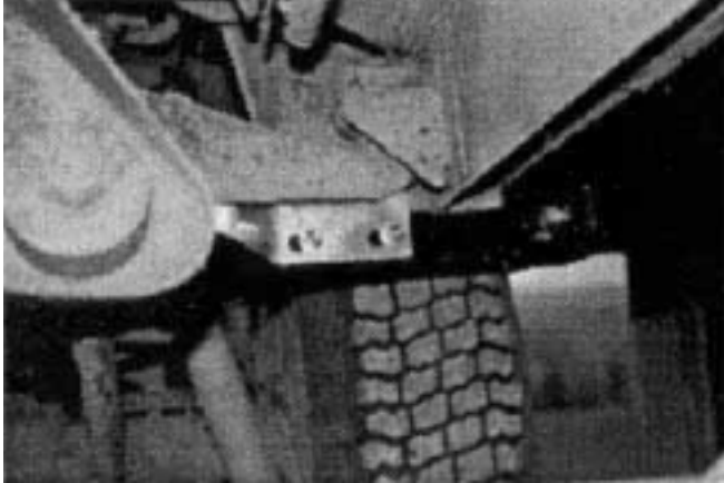
Fig. 8 Rear arm loosely attached to hanger
